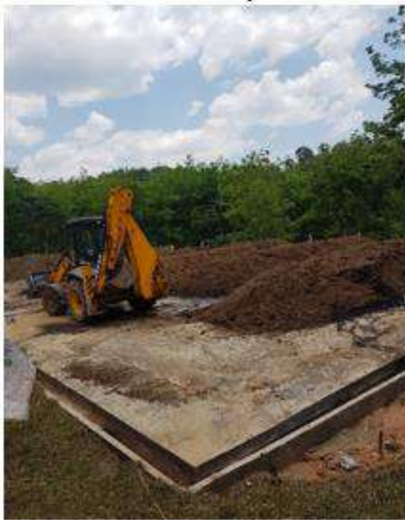
Out-door concrete pad for mixing and piling the composting materials as windrow piles
