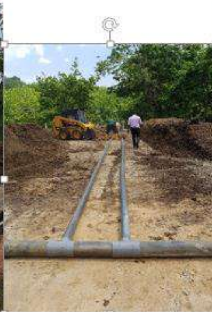
Arranging the pipes before piling the mixed materials
